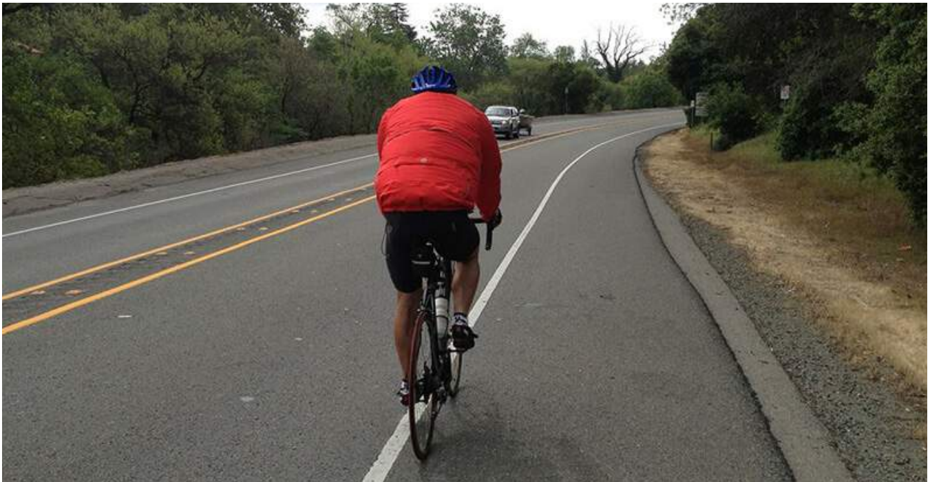
Example of Paved Shoulder
