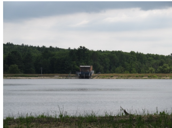
Figure 2. Brown Bridge Pond.
